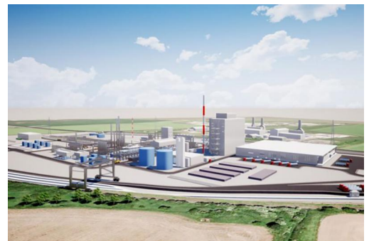
UK's Altalto plant will use the Fischer-Tropsch process to produce sustainable jet fuel from solid waste. Credit: Velocys
